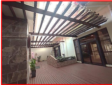
Figure 1 Existing Polycarbonate roof that needs to be remove.
