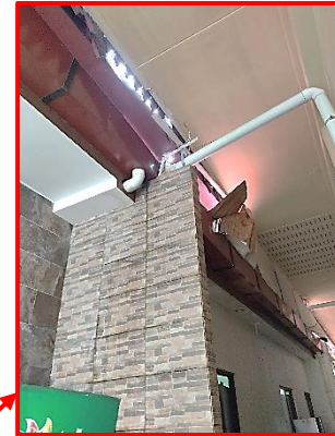
Figure 2 Damaged ICC building's steel gutter & PVC downpipe
